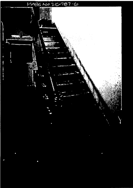
604 H Street NW, Washington, DC, Stairway from Second to Third Floors. 1988. Boucher, Jack. Historic American Building Survey, Library of Congress Prints and Photographs Division. http://hdl.loc.gov/loc.pnp/hhh.dc0913
